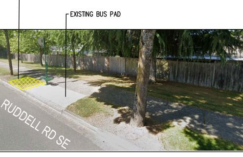
EXISTING CONDITION: BUS STOP PAD (APPROX. 14'X4.5'), 6' WIDE SIDEWALK, AND 4.5' PLANTER STRIP. INSTALL:10' WIDE PAD (APPROX. 10'X4.5') TO MEET THE LARGE PAD REQUIREMENTS. MATCH EXISTING TOP OF CURB AND SIDEWALK.
