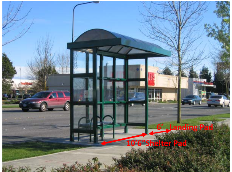
Cantilever shelter in planter strip.
