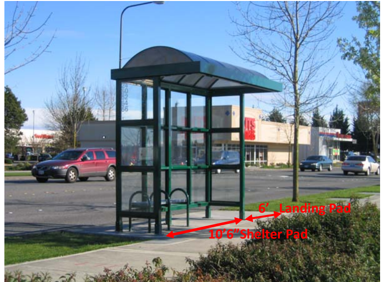
Cantilever shelter in planter strip.
