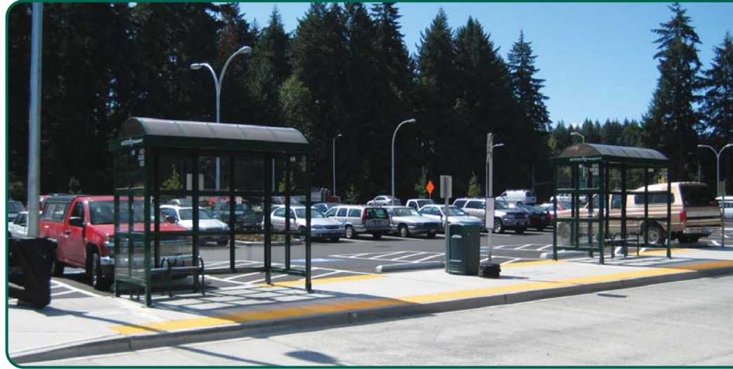
The newly expanded Martin Way Park & Ride lot, adjacent to I-5 exit 109 in Lacey, is the largest and most-used lot in Thurston County.
